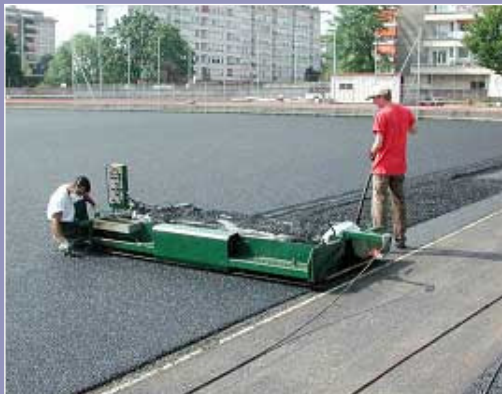
Elastic layer constructed in situ
